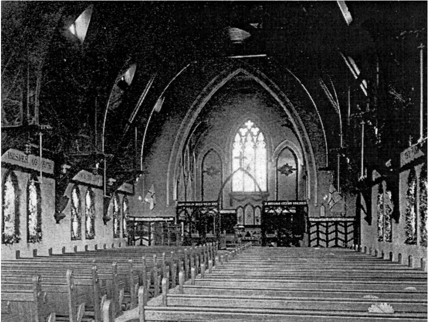
Original interior of church
