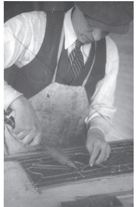
Soldering the lead came joints is one of the last steps in creating a stained glass window.
