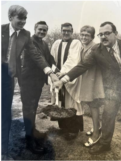
Groundbreaking for the first addition.
